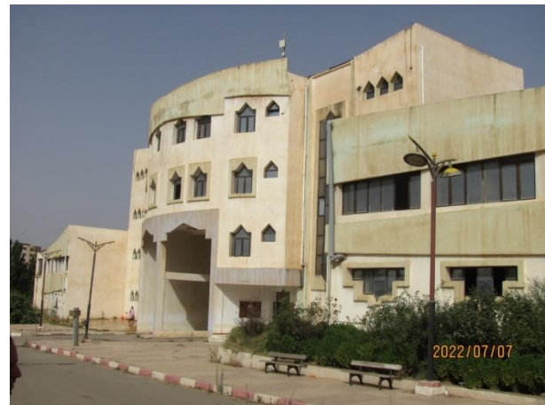
This building hosts the CUPAGIS equipment: PAGIS servers etc., VRC computer class and PASENSO office.
